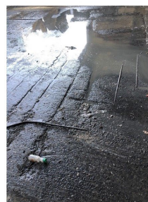
SOLID WASTE TRANSFER STATION
