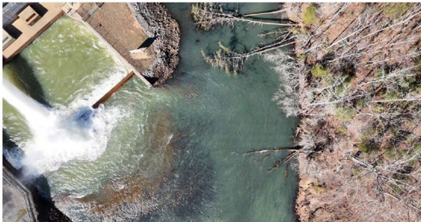
Site #1 - Waterway Debris Pictures
